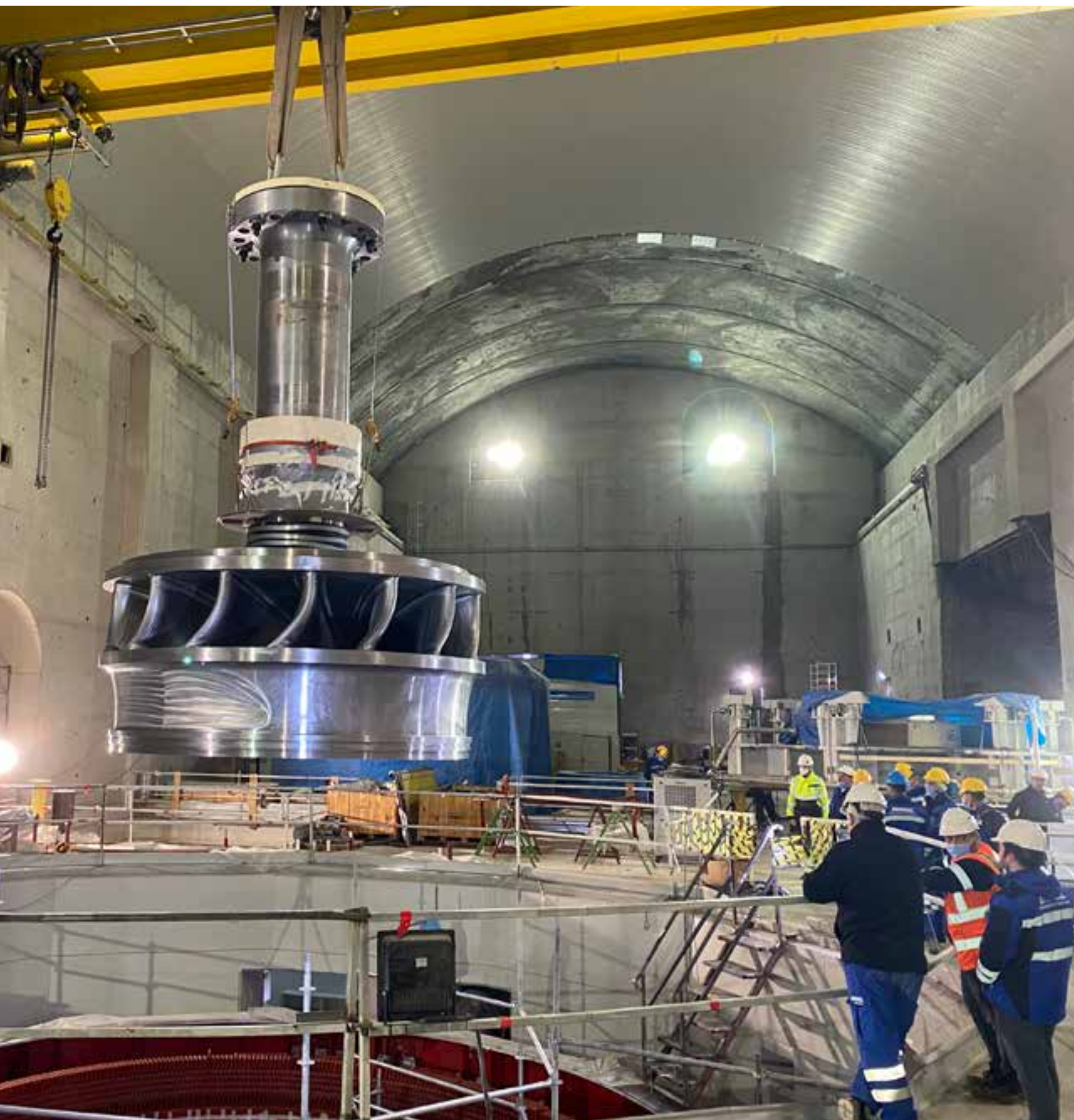
ANDRITZ Francis turbines power the Yusufeli hydropower plant in Türkiye, generating clean energy for 600,000 households through integrated water-to-wire technology.
