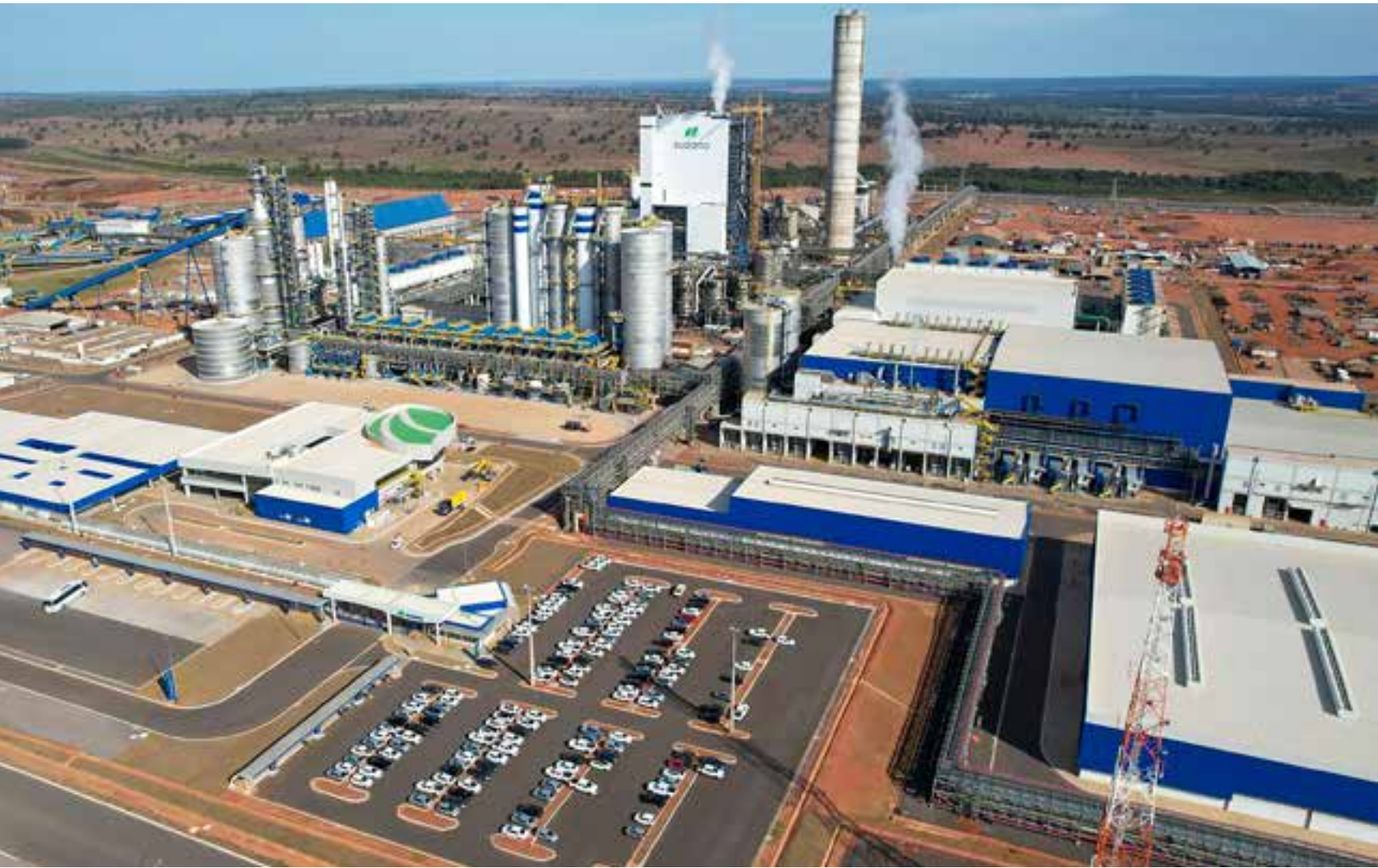
Suzano's state-of-the-art pulp mill in Brazil, featuring ANDRITZ's comprehensive fiber production and chemical recovery technologies, including the world's largest single fiberline
